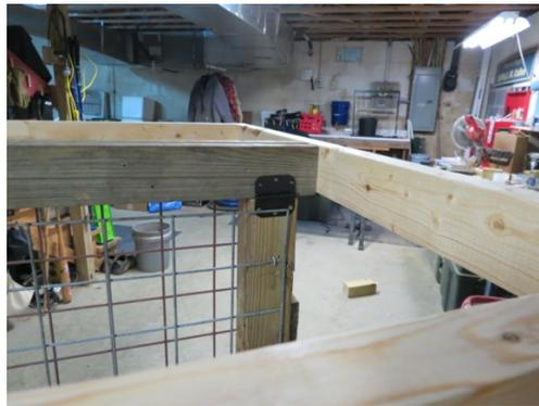
Step 4 – attach the hinges. Here is where you need a second person to hold the frame steady unless you have a device to secure it for you. We used the woodscrews here as well.
